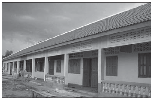
Almost completed preschool in late June
