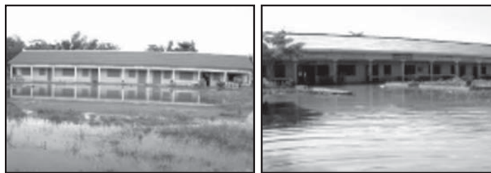
Flooded secondary school (left), library, offices and preschools.
